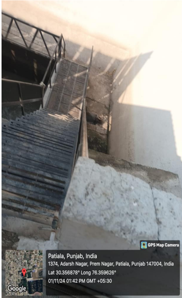
FIGURE 2. BAR SCREEN & COLLECTION CHAMBER
