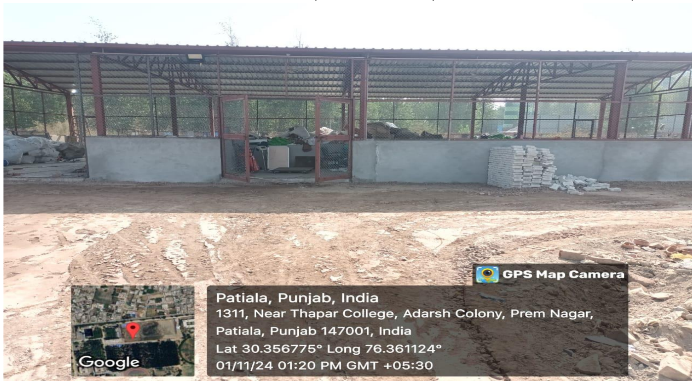
FIGURE 1. MRF FACILITY NEAR STP PLANT
