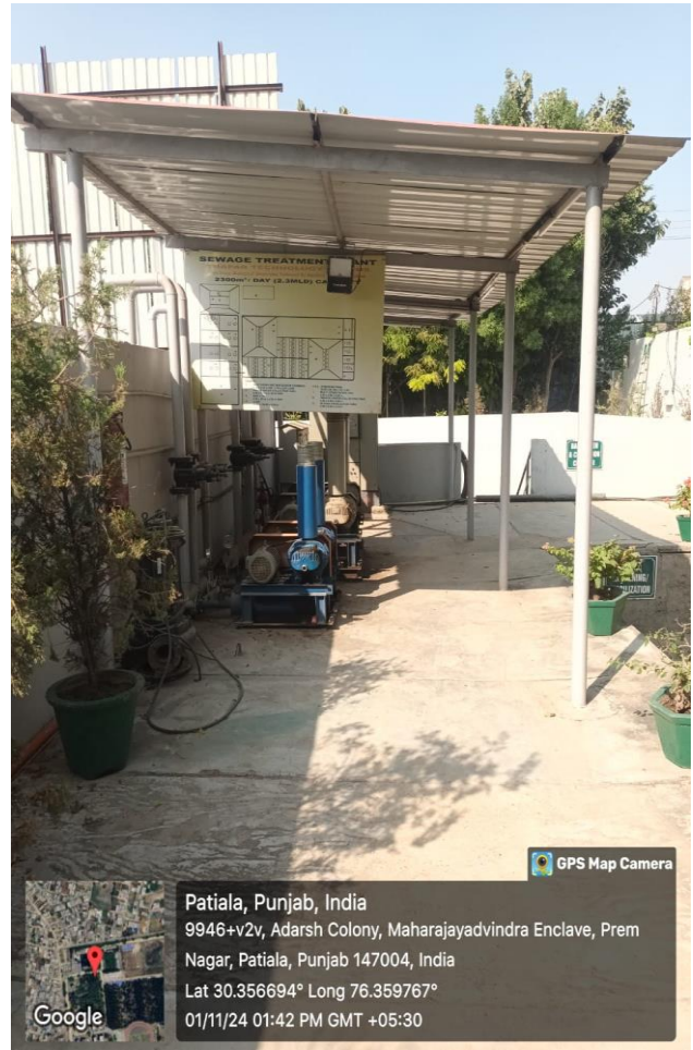
FIGURE 3. STP PUMP SYSTEM
